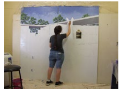
Painting building, under canopy
